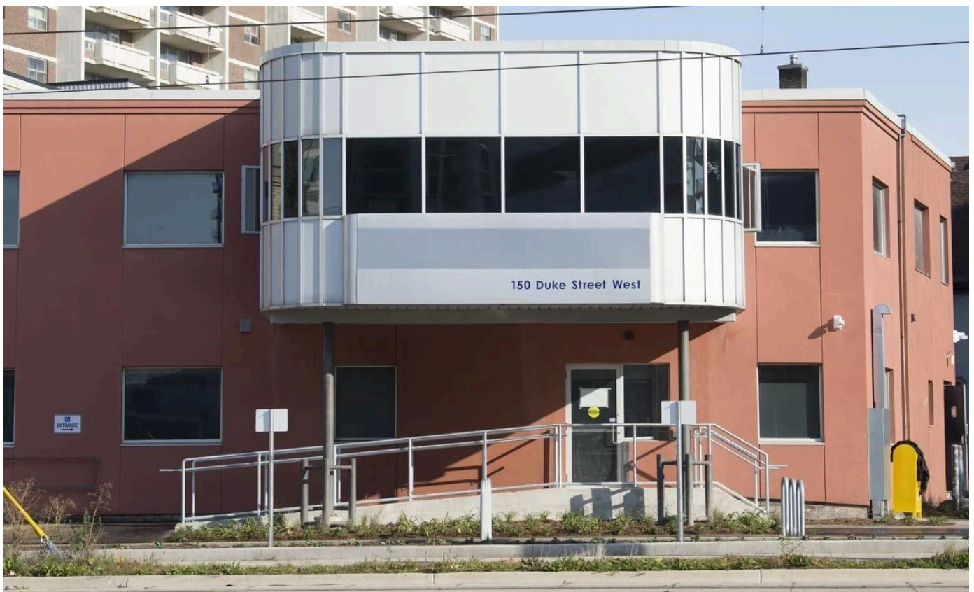
The consumption and treatment services site at 150 Duke St. W. in downtown Kitchener.
